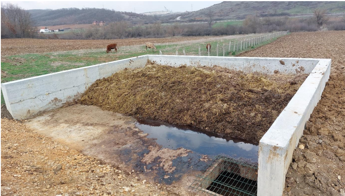
Manure heap on a sealed concrete surface with walls on three sides to prevent seepage of nutrients into the soil. Seepage is drained and collected via a channel grid. © Bettina Schwarzl
